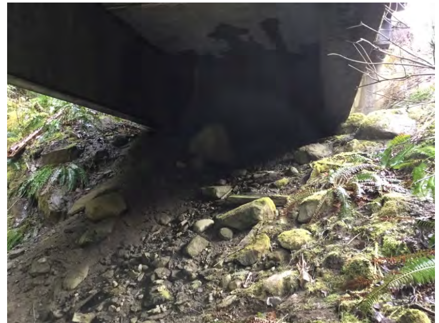
Left Bank Abutment when facing downstream
