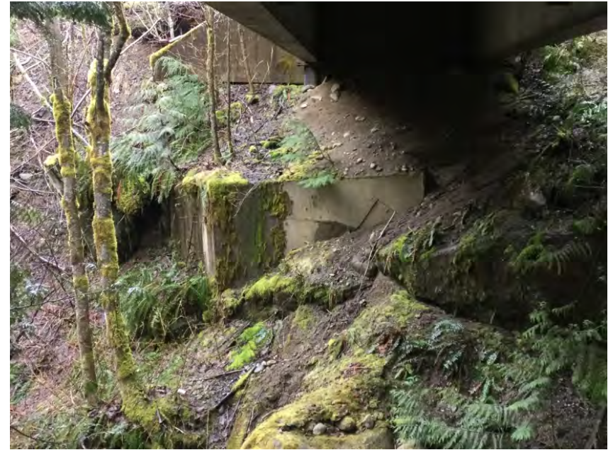
Right bank CIP place sloped to downstream
