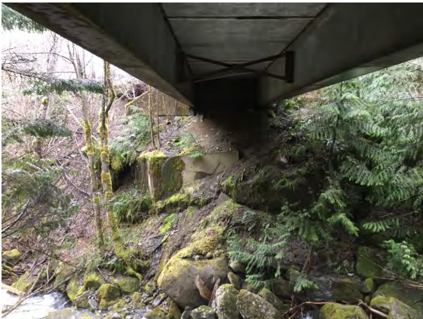
Right Bank Abutment when facing downstream
